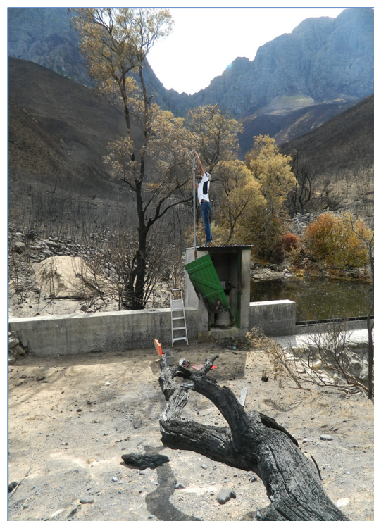
SAEON staff remove a melted antenna from the Langrivier gauging weir hut at Jonkershoek after a wildfire in March 2015
